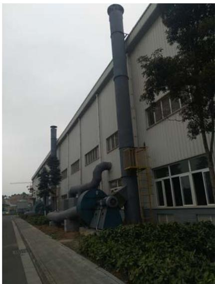
铸造车间制芯、浇注、熔炼排气筒及净化设施
